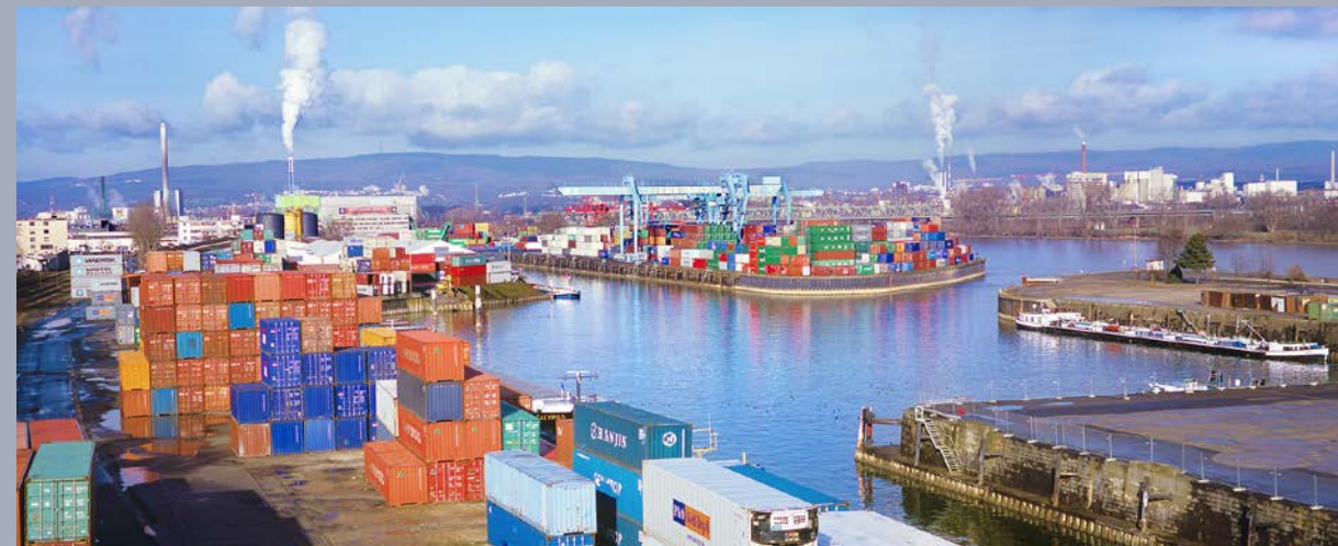
2008 RELOCATION THE CONTAINER PORT IS MOVED FURTHER DOWN THE RHINE TO THE INDUSTRIAL PORT.
